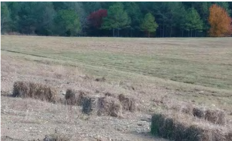
LF4-03: BMPs were in place to fix rills noted in previous inspections and prevent erosion.
